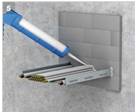
5 After the insertion of the bricks close all joints with ROKU® FL Sealant.
