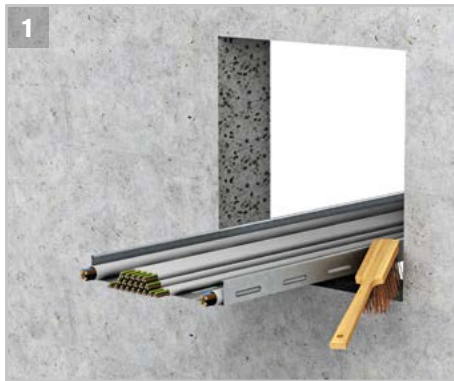
1 Clean the aperture and remove all loose parts.
