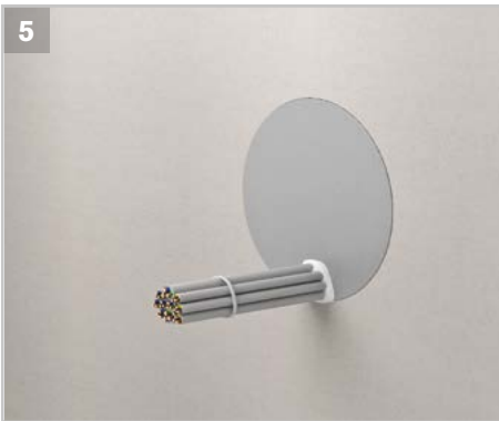
5 Check the sealing.
